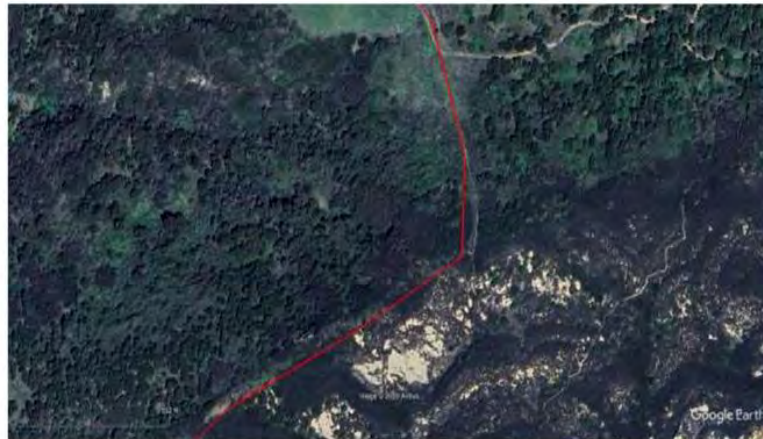
Fig. 1a. 2,000-foot long section of pipeline route (red line) in Gaviota State Park on 18 April 2025.
