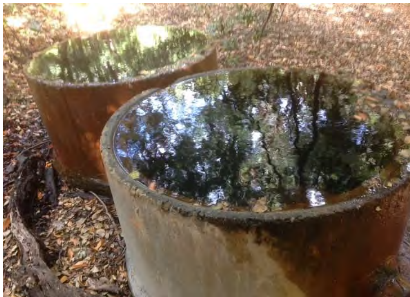
Figure 283. These cisterns along Arroyo Burro Trail near San Antonio Creek are filled with water from a streambed diversion. Brian Trautwein. June 2020.
