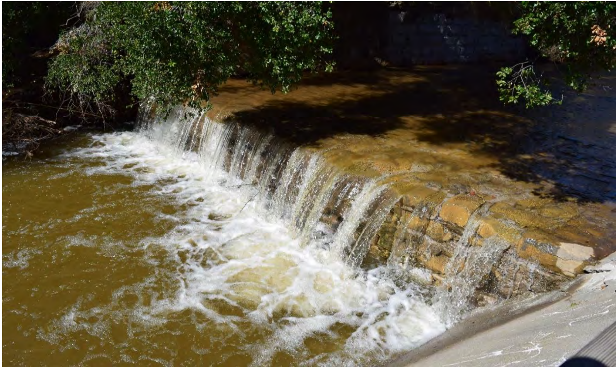
Figure 16. This check dam on Maria Ygnacio Creek below the UPRR bridge inhibits steelhead migration. February 6, 2019.
