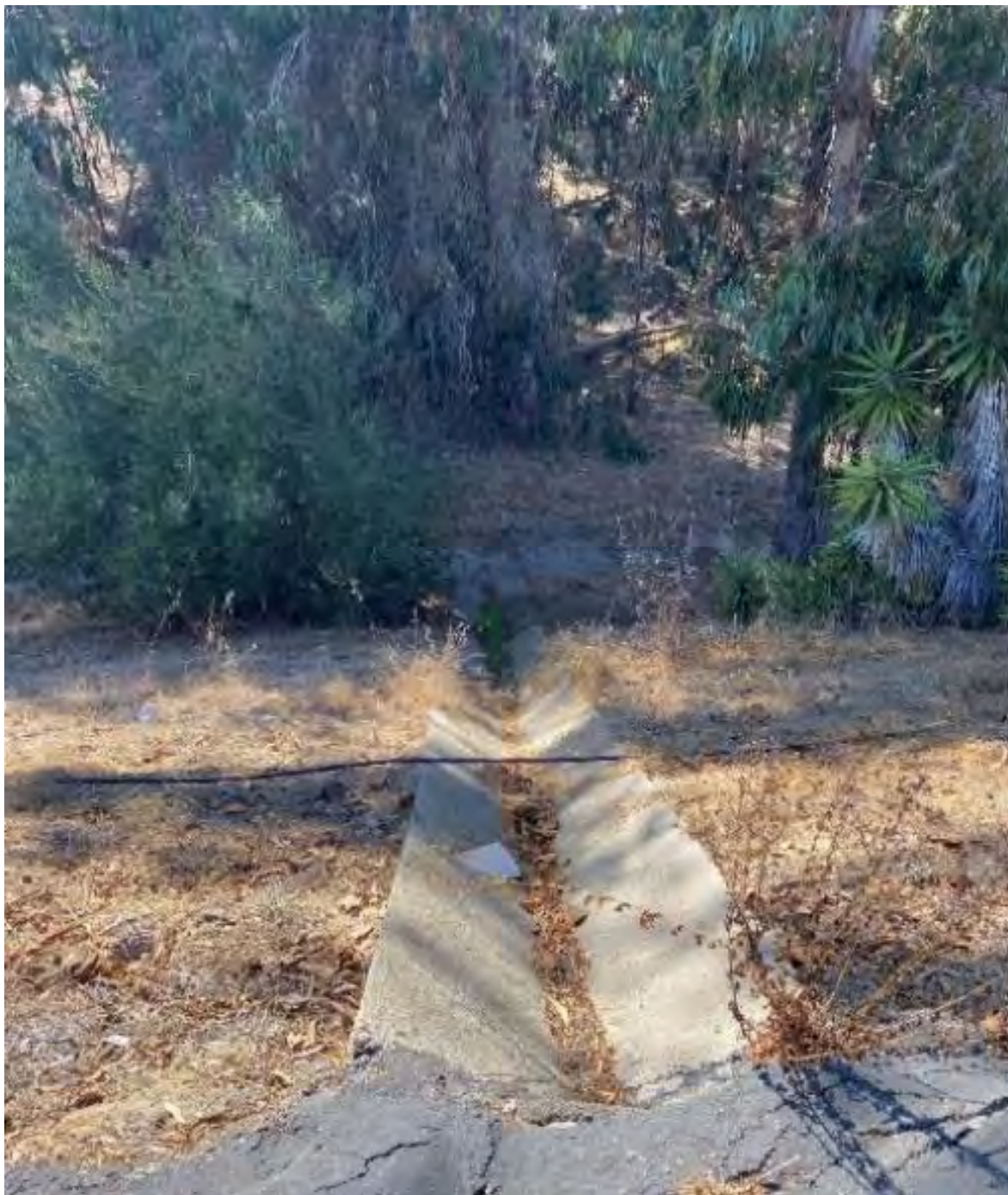
Figure 74. A concrete-lined storm drain directs parking lot runoff into the tributary without any opportunity for infiltration. Brian Trautwein. October 2020.
