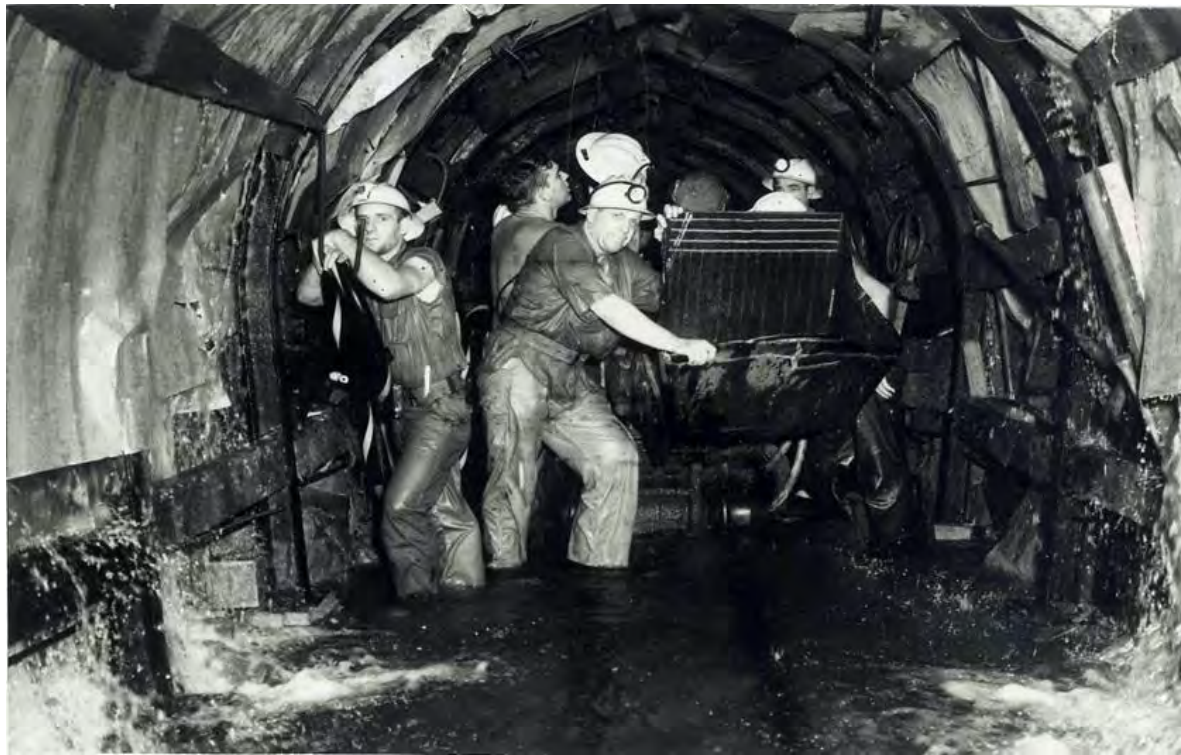
Figure 9. Workers constructing Tecolote Tunnel with groundwater infiltrating the borehole. Cachuma Operations and Maintenance Board, 1954.
