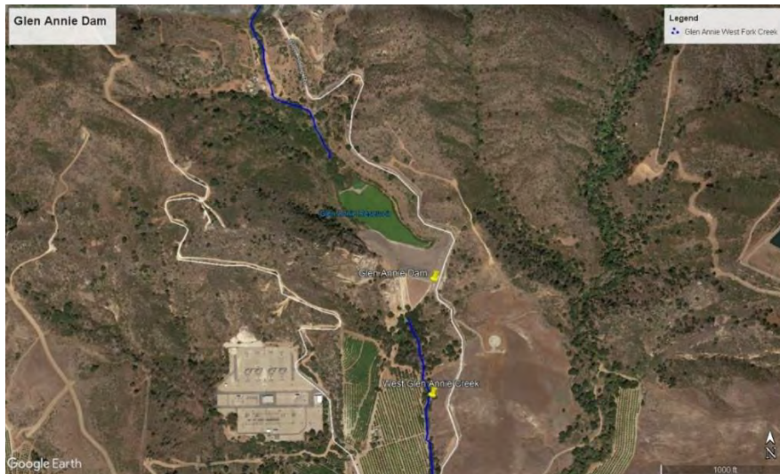
Figure 8. Glen Annie Dam and Glen Annie Reservoir on West Fork Glen Annie Creek. Google Earth. 2014.
