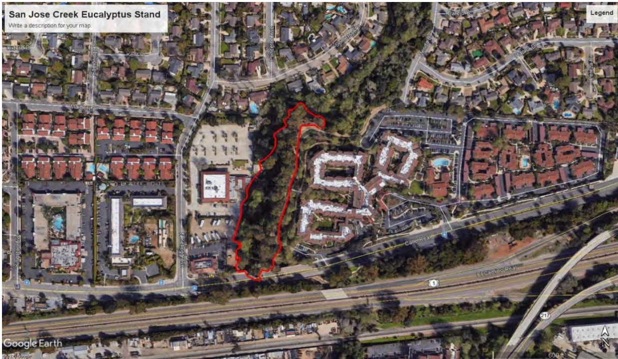
Figure 219. This substantial eucalyptus grove once served as a monarch butterfly overwintering site and turkey vulture roost. It creates a fire hazard near the Maravilla Assisted Living Community. Google Earth. 2019.
