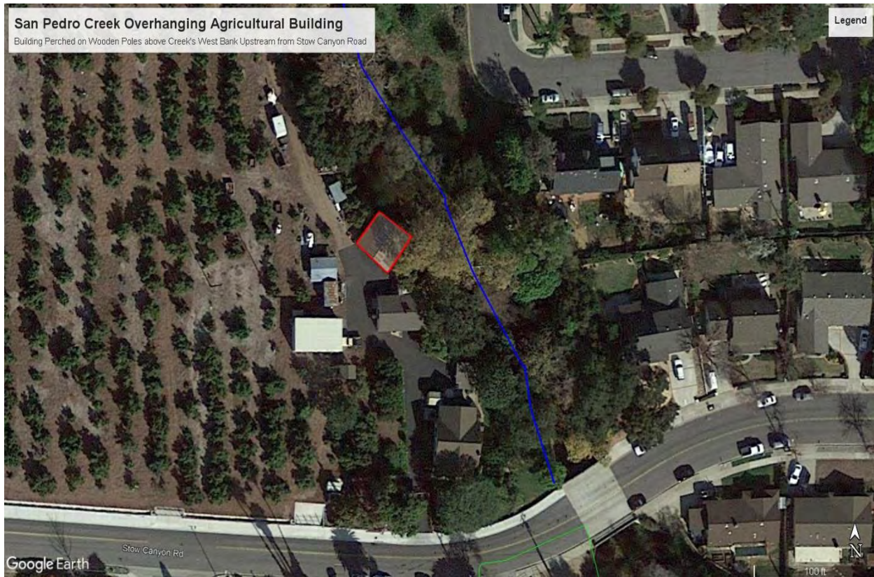
Figure 129. An agricultural storage building (outlined in red) is perched over the west bank of San Pedro Creek (blue line). Google Earth 2019.
