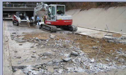
Demolition of the Upper Channel of Mission Creek Photo Courtesy of the City of SB Creeks Division
