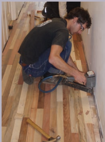
Installation of EDC's new hardwood floor.
