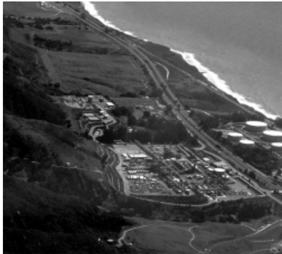
Gaviota Oil and Gas Facility
