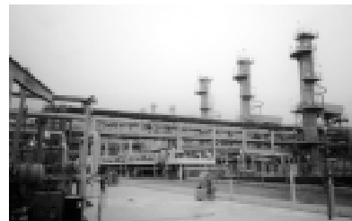
The County is re-evaluating the status of the Gaviota consolidated facility.
